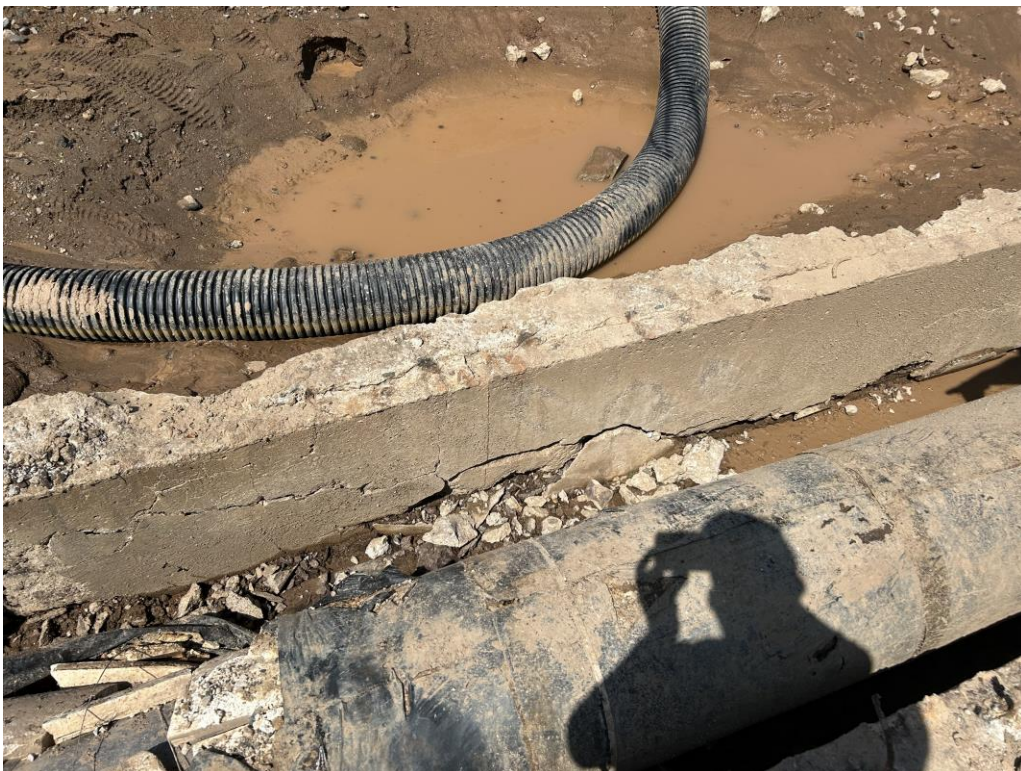
Figure 2: Steam Tunnel Wall: West Wall
