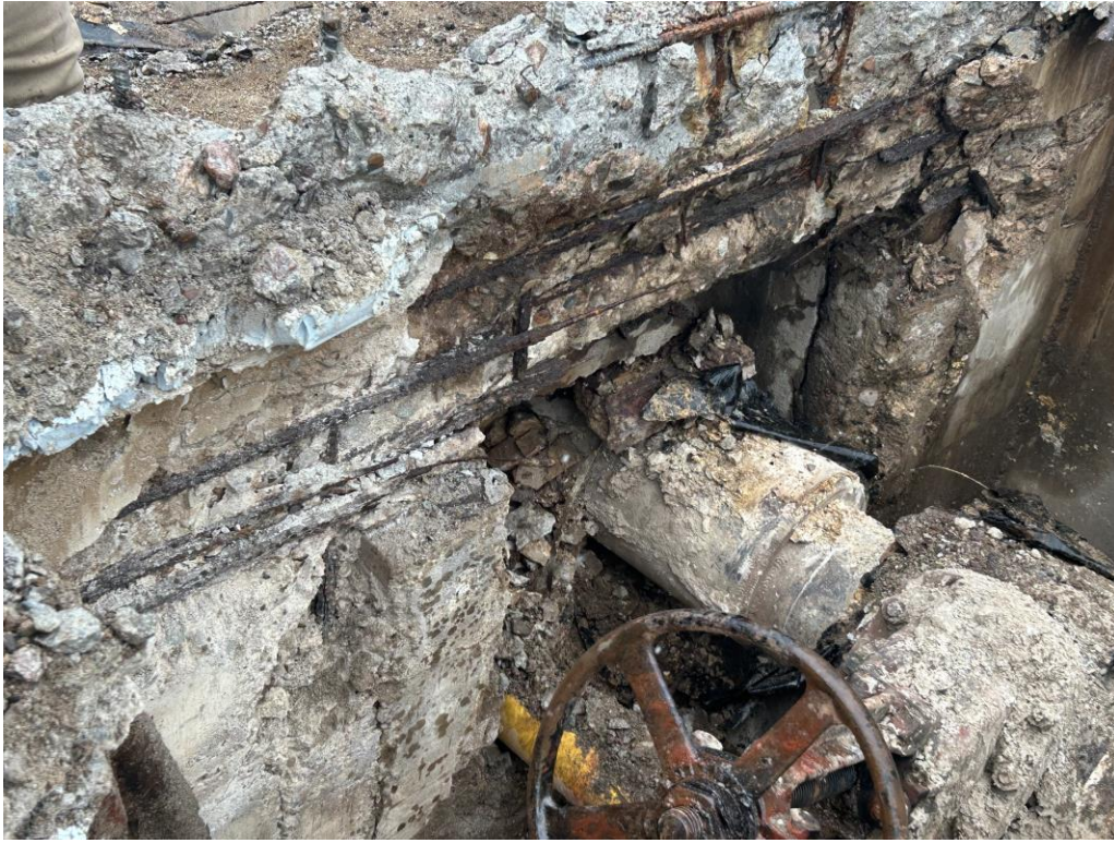
Figure 1: 9th Avenue Vault: North Wall
