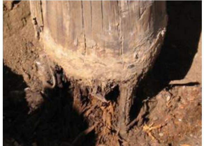
PICTURED: GROUNDROT AND HOLLOW POLE EXAMPLES BEING REBUILT
