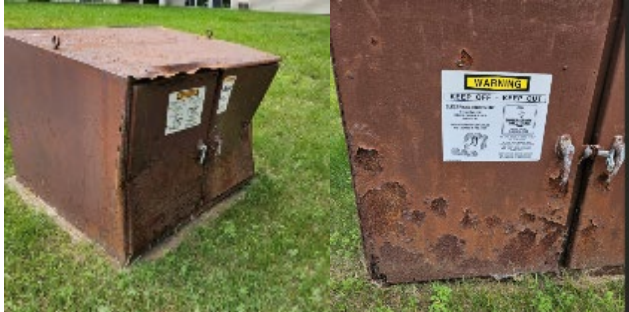
PICTURED: MECHANICAL DAMAGE ON FDR 15 CABINET
