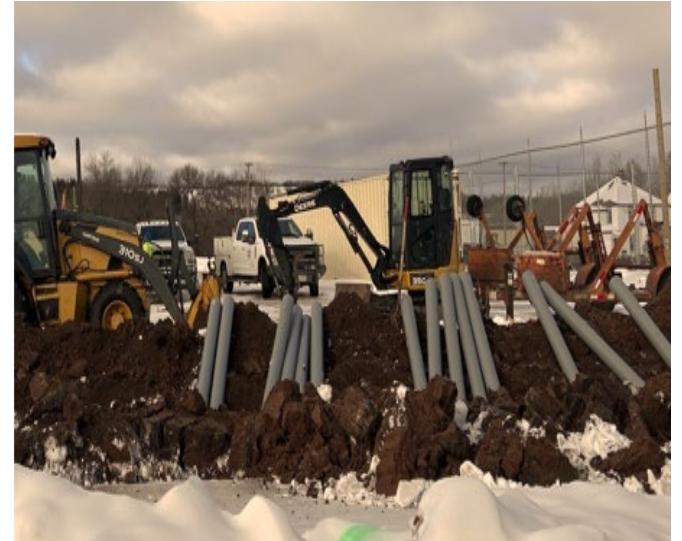
PICTURED: CABLE AND CONDUIT EXCAVATION AT FIRST AVE SUB SITE
