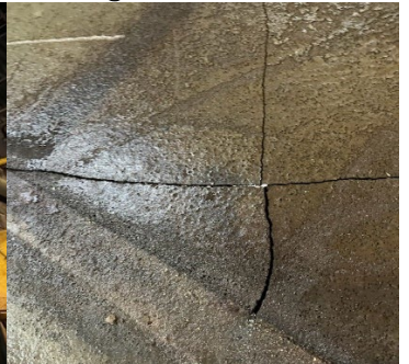
Damage Under #4 ID Fan
