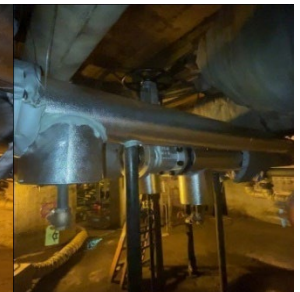
Cond't Valve Installation
